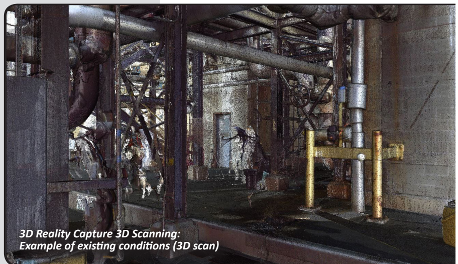
3D Reality Capture 3D Scanning: Example of existing conditions [photo]
